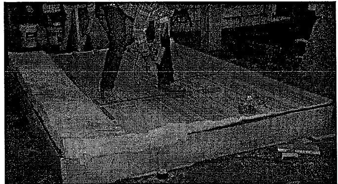
Figure 7: Fastening Exterior to Purlins
