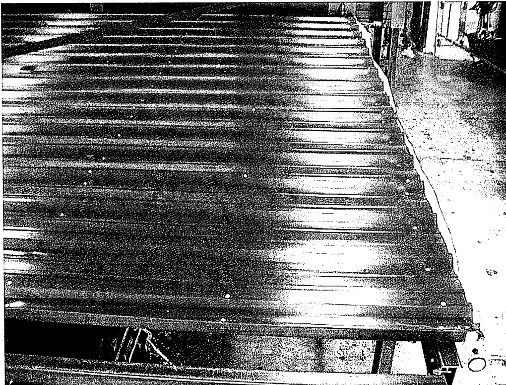
PHOTO 4 View of the panel fasteners at end and intermediate supports. (DSC00069)
