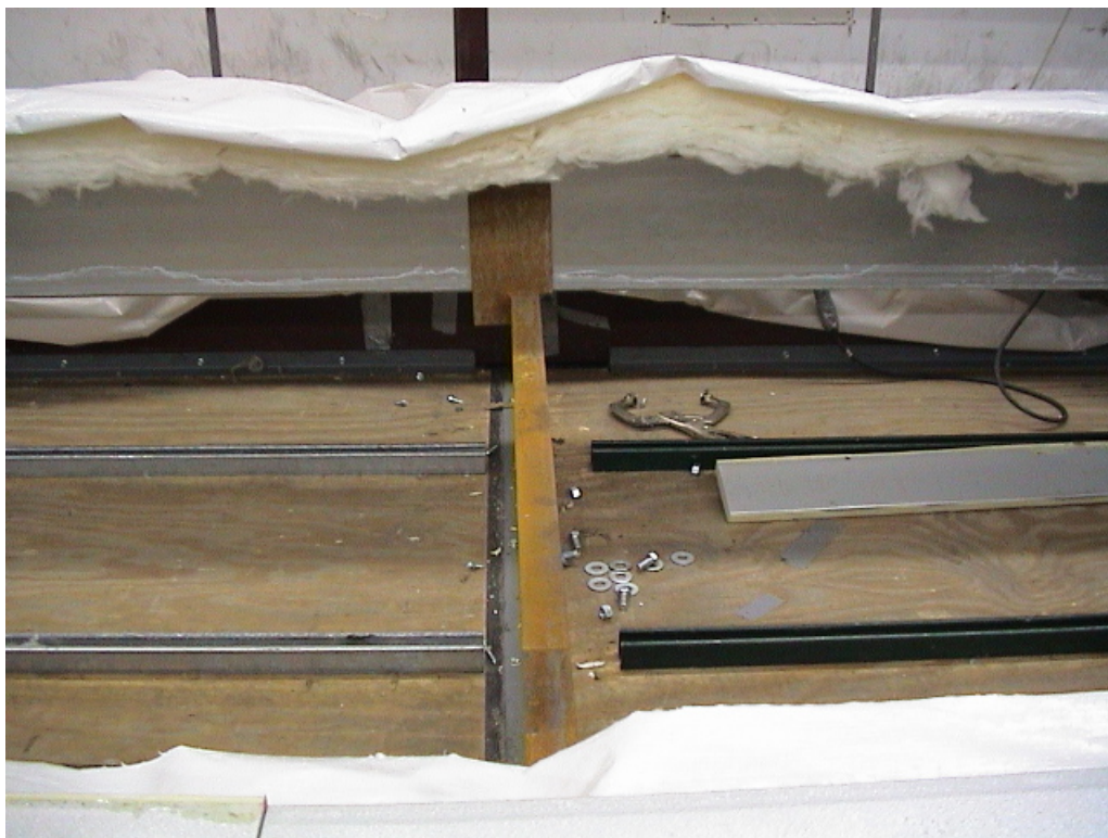
PHOTO 13 View of attachment of retrofit bracing at midspan. (DSC00128)
