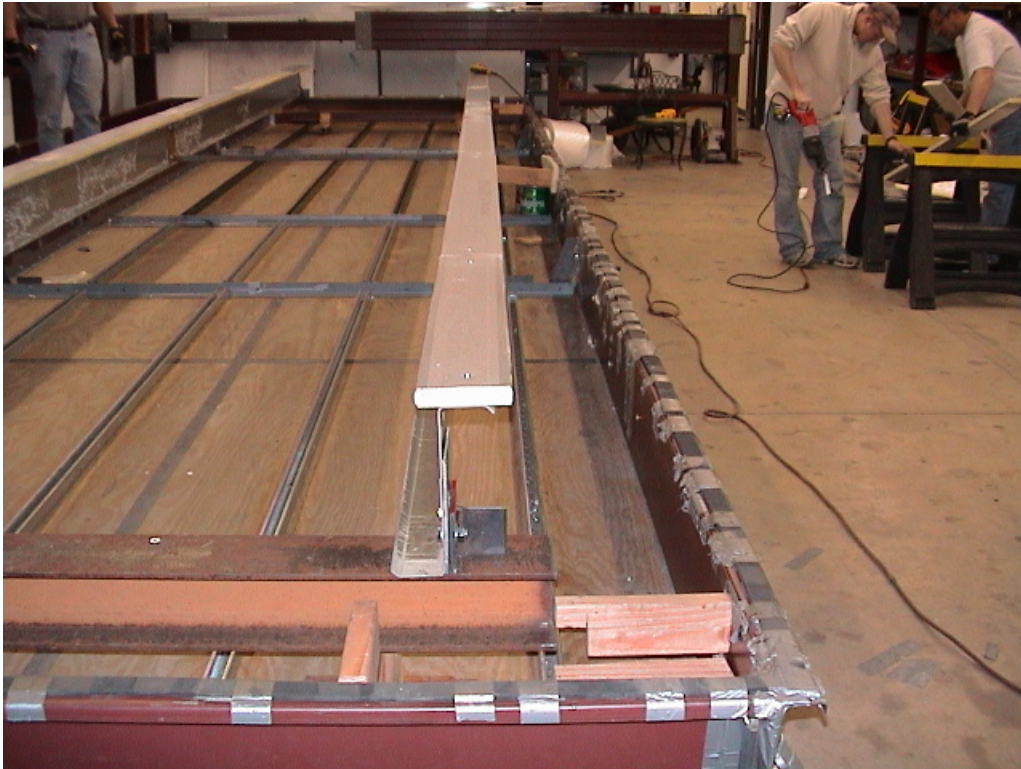
PHOTO 19 View of the Sealed 'N' Safe™ thermal block attachment to purlin without 3" thick insulation. (DSC00025)
