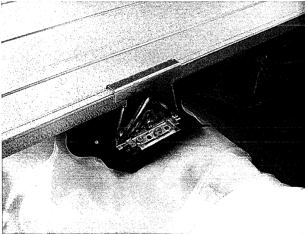
PHOTO 4 View of the panel clip attachment. (DSC00087)
